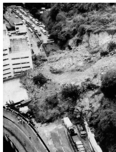
Fig. 3. Landslide debris on 13 August 1995.
