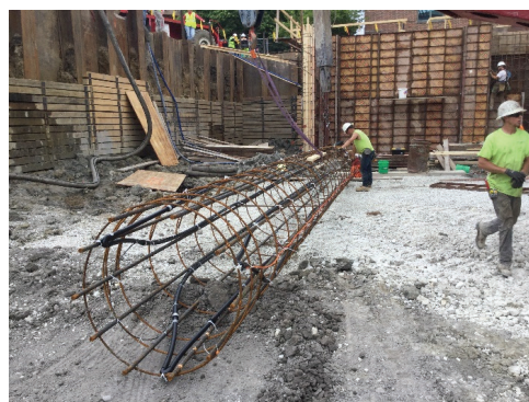
Fig. 5. Energy foundation construction at the University of Illinois
