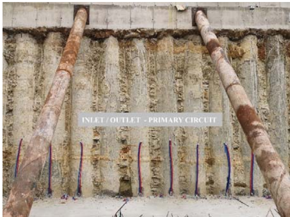
Fig. 7 Inlet and outlet of primary circuit at the bottom of excavation level at the extraction stage
