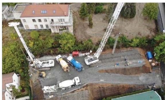
Fig. 6 Execution of the 1000 mm energy piles
