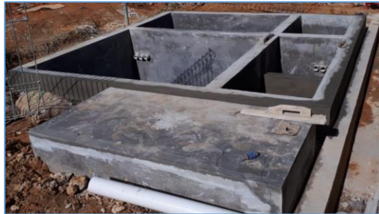
Fig. 4. Cooling water treatment
