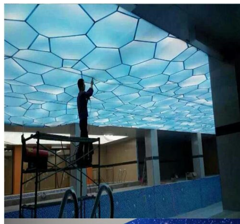
Figure 3. Actual application effect drawing of stretch ceiling.
