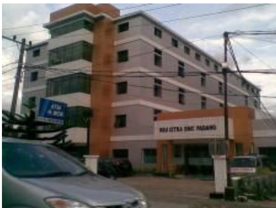
Fig. 3. Side view of block D building
