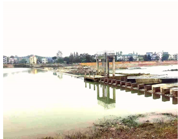
Fig 1. Leakage at the intake
