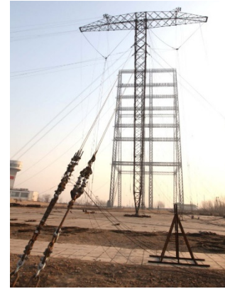
Fig. 5. The site of the full-scale test
