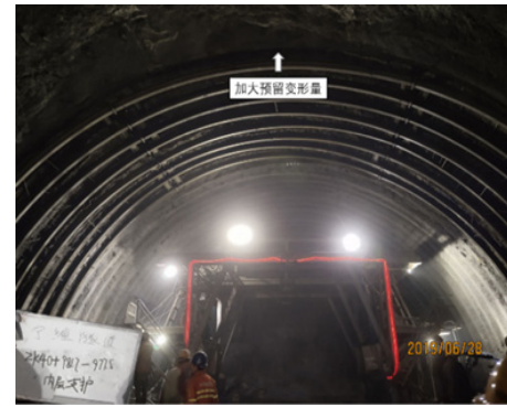
Fig. 9 Increasing Reserved Deformation of S3 Support
