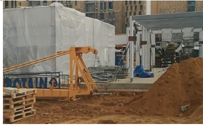
Fig.1. Building block modules erected in building conditions.
