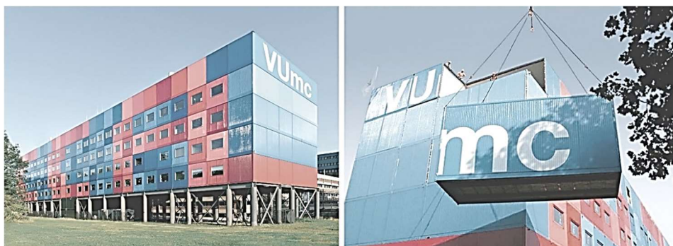
Fig. 10. Design and assembly of modular containers [19].
