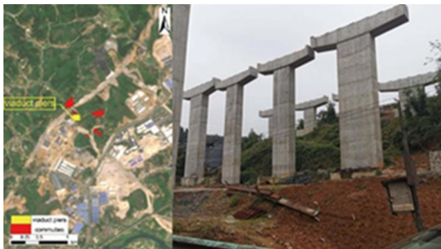
Fig. 2. The study area and the downstream viaduct piers
