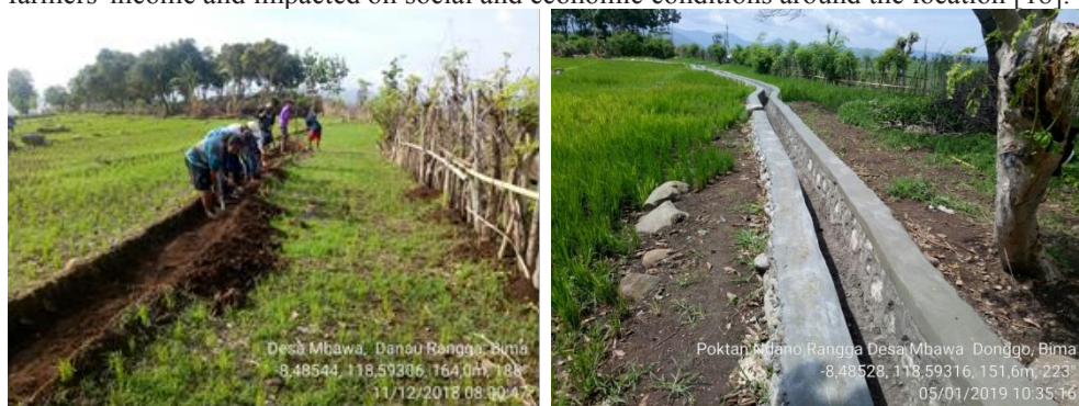
Fig. 1. Channel condition before (A) and after (B) rebuilt
