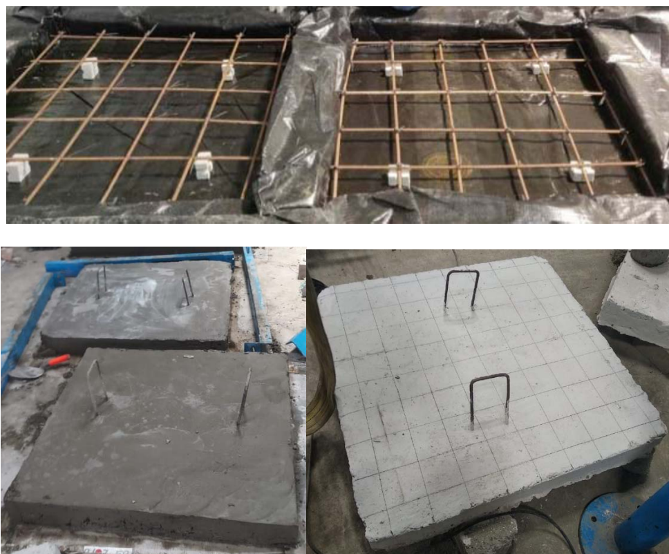
Fig.4. Casting of slabs
