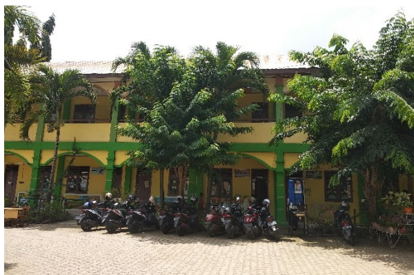
Fig 4 (a). Meuraxa's school building
