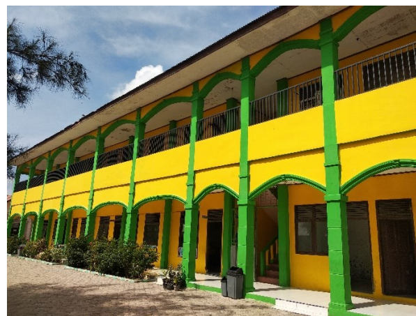
Fig 3 (a). Kutaraja's school building
