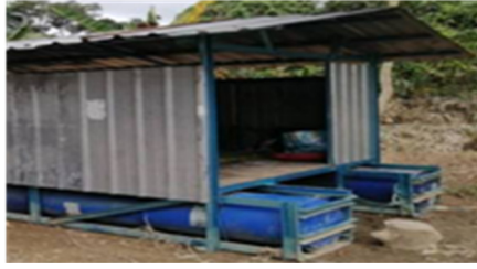
Fig. 2. An Isolate – Self-reliance as opposed to dependence during disaster: A man from Temerloh created a RM1000.00 floating hut for her mother. The destructive impact of 2014 flood and floating fish cage idea motivated him to be prepared for 2020-21 flood. [16]
