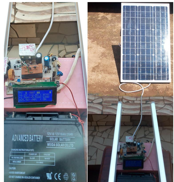
Fig. 9. Experimental setup of DAK with PV Module
