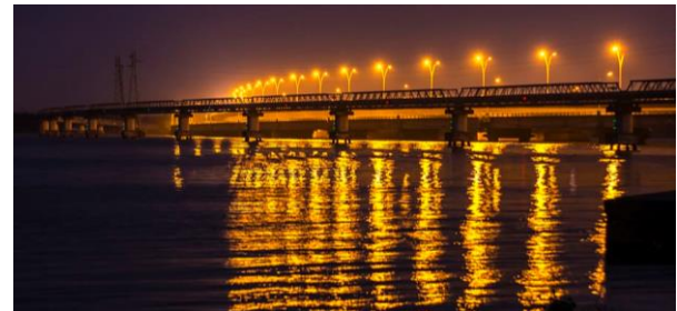
Fig. 2. The second bridge over River Wouri by night [12]
