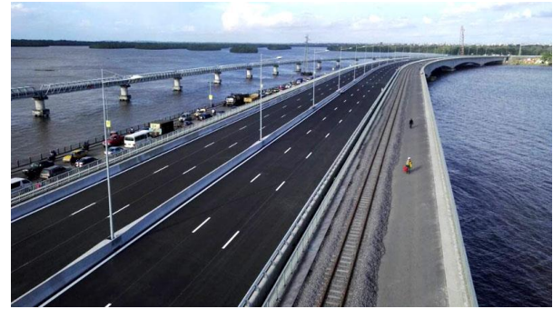
Fig. 1. Second Bridge over the River Wouri [11]
