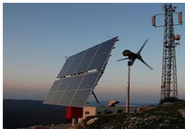
Figure 1: typical off-grid hybrid PV-wind-diesel powered mobile base station [2].
