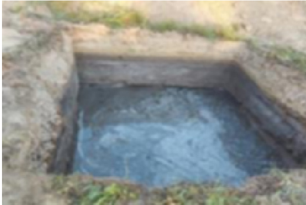
Fig. 1. Soaking the base of the soil cushion.
