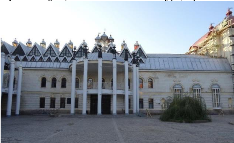
Fig. 1. General view of the surveyed building.
