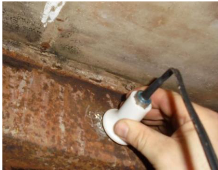
Fig. 9. Determination of the actual wall thickness of sections of steel structural elements by the contact echo pulse method using the TT-100 device.
