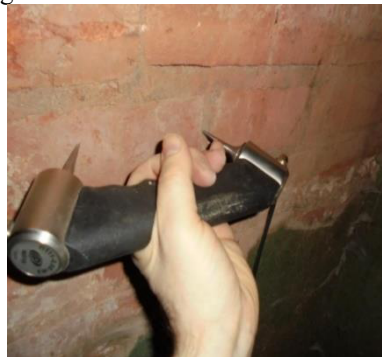
Fig. 6. Determination of brickwork strength by ultrasonic pulse method.
