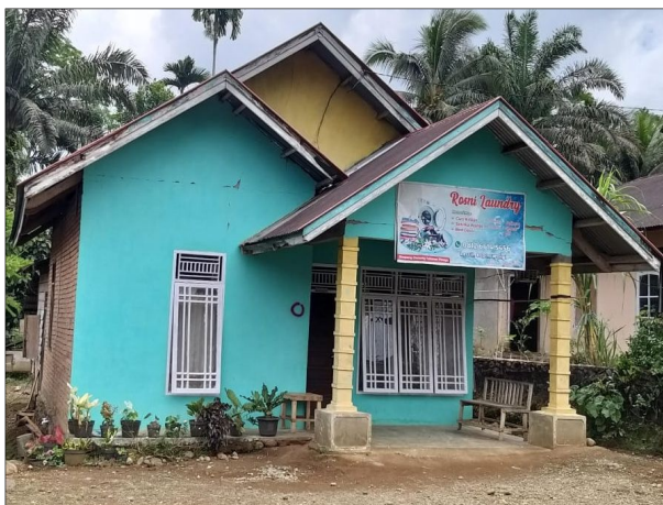
Fig. 2. Lite damaged house.
