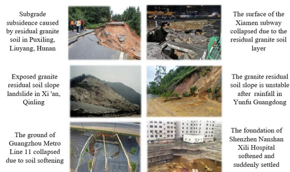
Fig. 1 Geological hazards of unsaturated granite residual soil [2]
