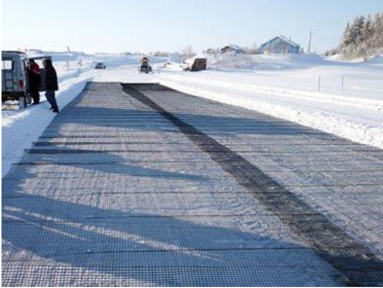
Fig. 1. Example of ice road reinforcement ( https://miakom.ru/tekhpodderzhka/primeneniye-materialov/primeneniye-steklosetki-geo-st/armirovaniye-ledovykh-pereprav/ )
